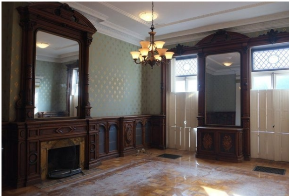
A principal parlor, with twin carved overmantel mirrors, a marble mantel, and parquet flooring.
